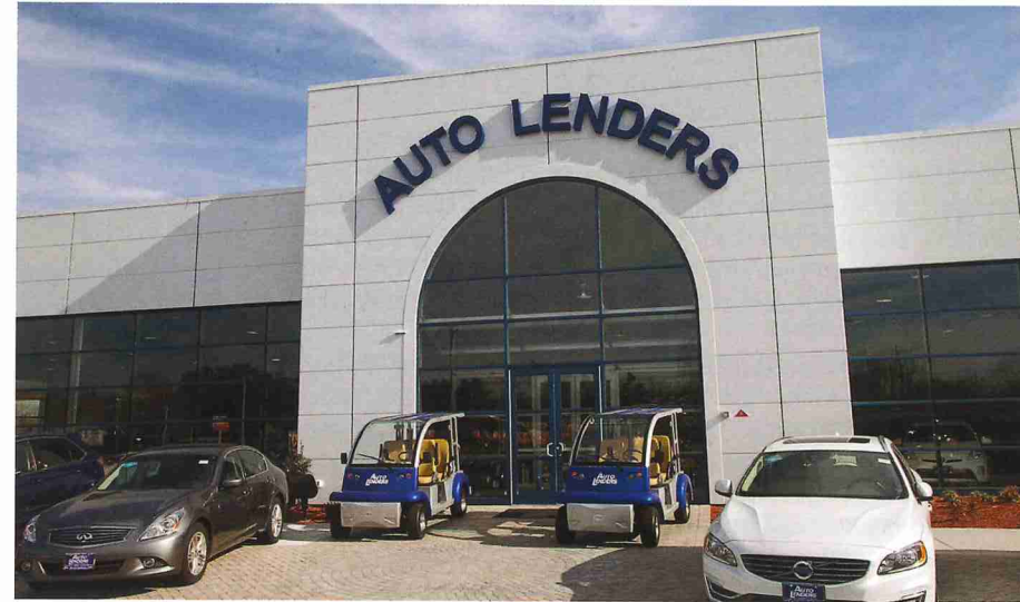
The 30,000-square-foot facility uses pre-finished metal panels and plenty of glass.
