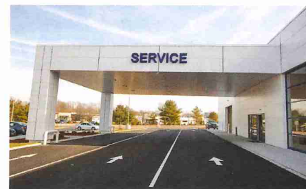
A three-lane drive-through service area.
